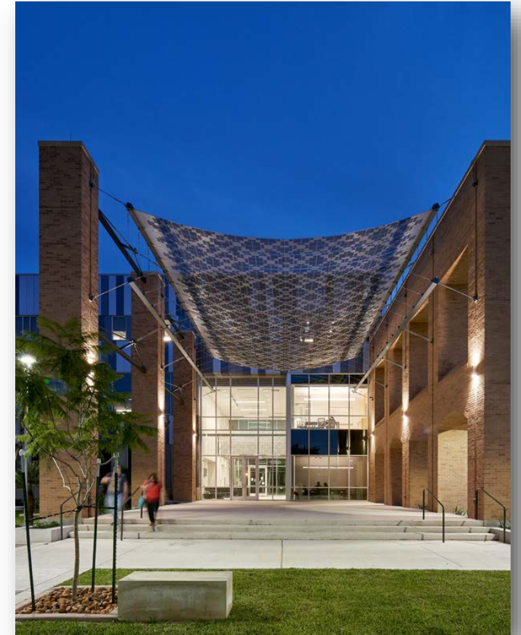
University of Texas Rio Grande Valley, Interdisciplinary Engineering and Academic Building
